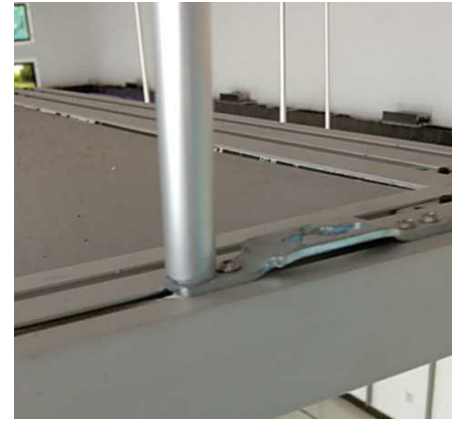
Suspended detail WATERPROOF CLOUD MEDIA FRAME
